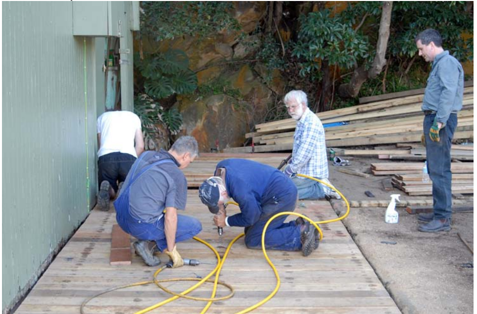
Drilling for the many hundreds of screws to hold it all in place
