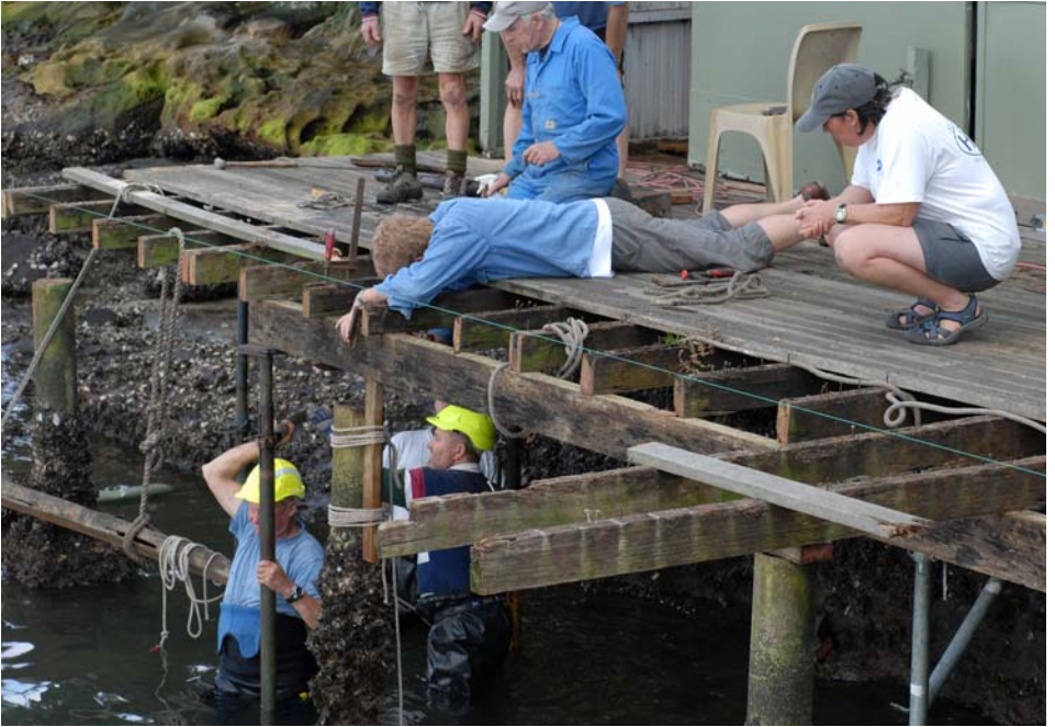
The in-water crew adjusting levels
