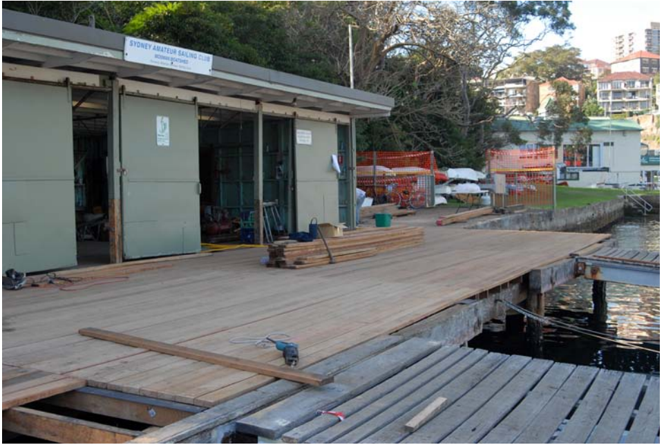
The new deck nearly finished
