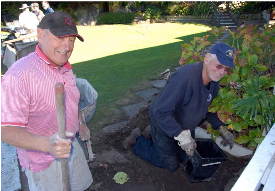
Practical plumbing in the garden (above)
