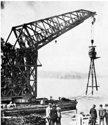
The floating crane Titan about to place the mast on Bradley's Head in 1934
