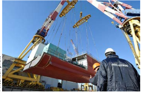
Placing the first block for the new Costa cruise liner
