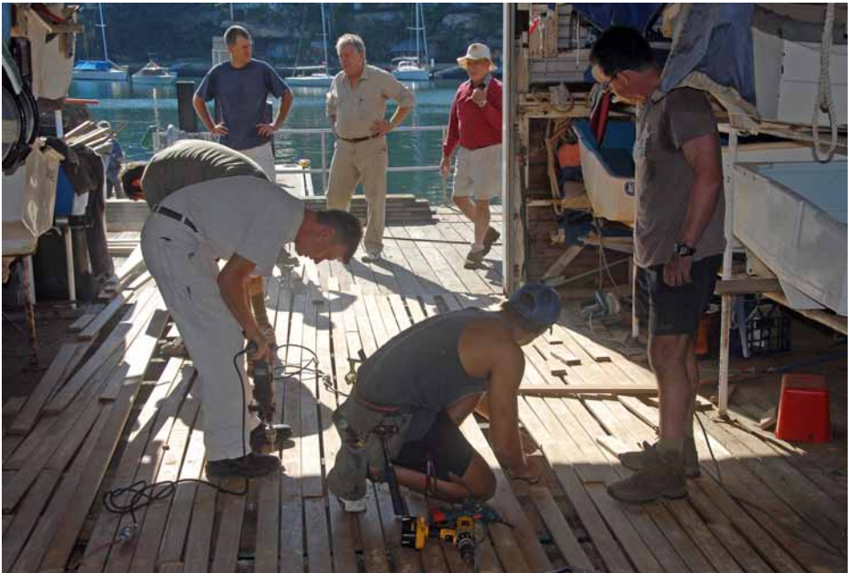
Welcome repairs to the boatshed floor (below)
