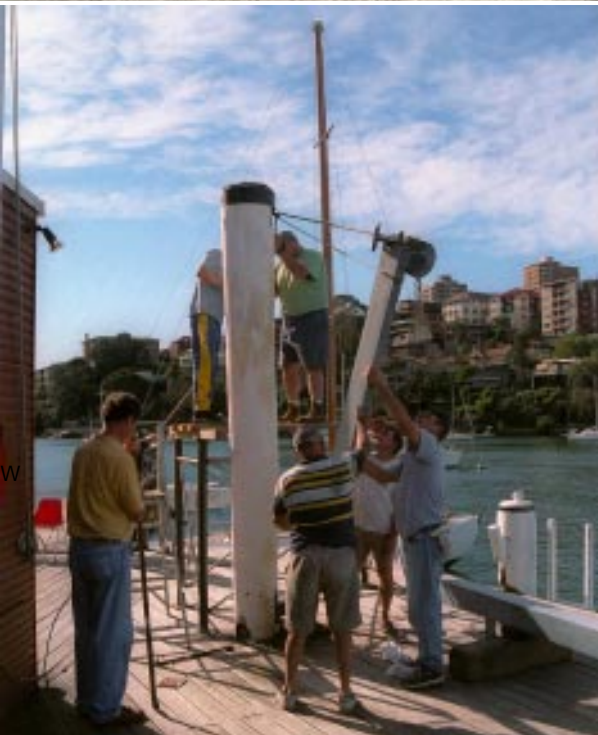
Augmented by further volunteers, the team removes the remaining steelwork (left)
