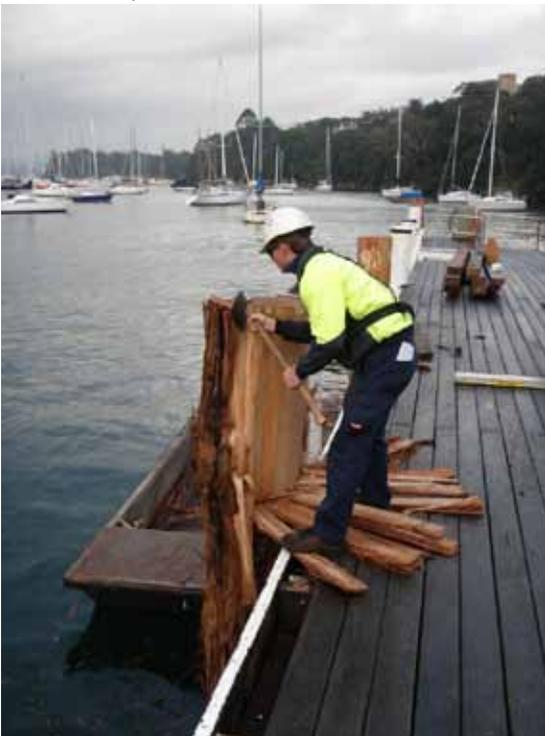
Placing a new free-standing pile off the SASC Wharf (above). Good progress was made in July on the repairs to the wharf and piles. The work should help hold everything together for a good few years to come
