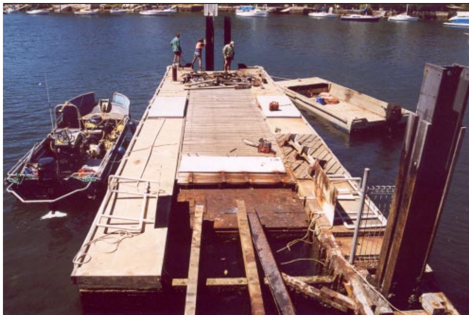
4 November — Demolition of the old pontoon underway (above)
