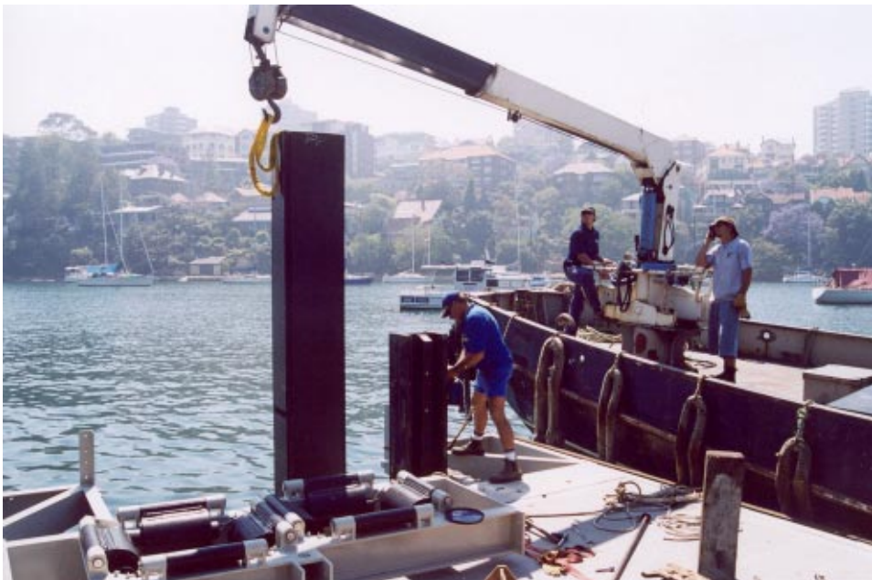
8 November — Fitting new HDPE sheaths to the existing steel piles (below)
