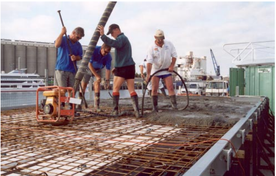
18 October — Pouring the concrete. About 18 cubic metres were required (below)
