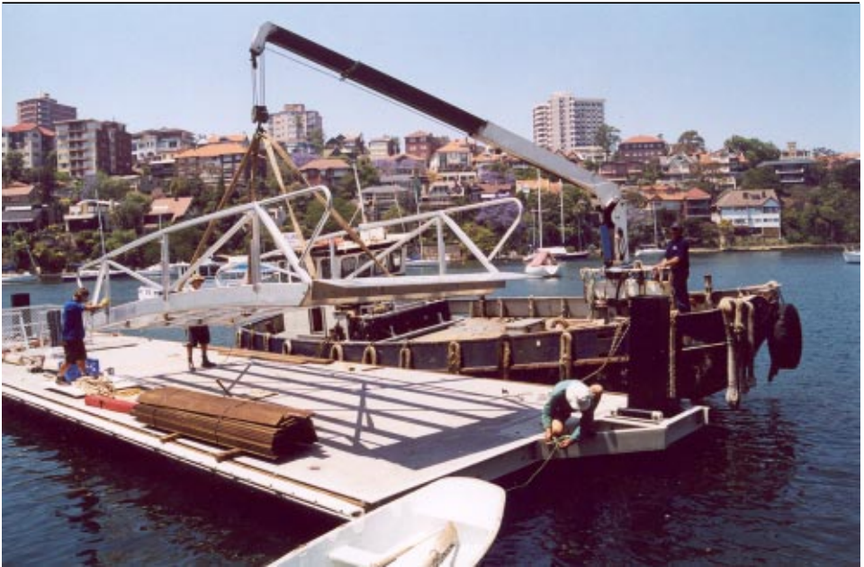
8 November — Lifting the new ramp into position (above)
