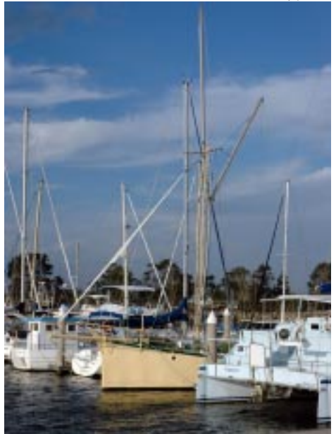
It looks as if someone forgot to trim the piles! Actually, they have to be that high at the new South Grafton Marina to ensure that the pontoons don't float away during a flood. The top of the piles is the same height as the levee banks. Luckily we don't face that kind of challenge in Mosman Bay — although there is global warming to consider
