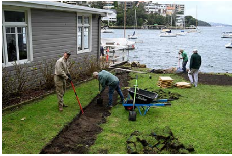
Excavations for the new path
