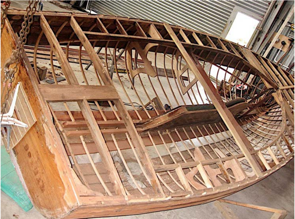
Rebuilding a derelict 18-footer
