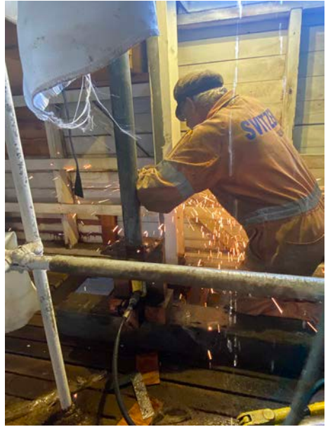
Cutting the column
