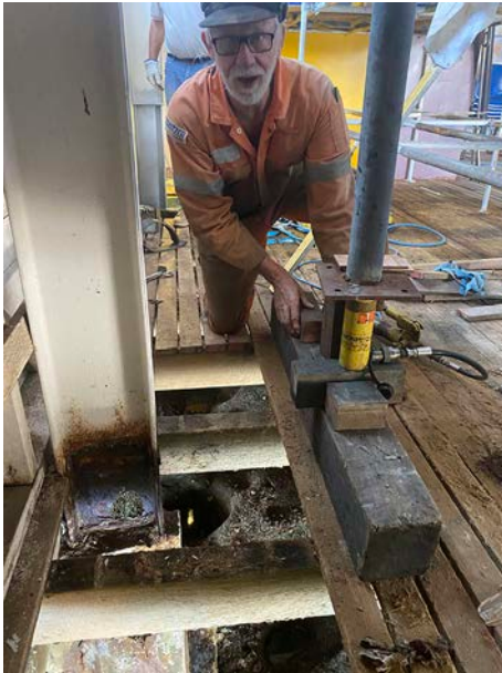
Trevor Cosh shoring up the boatshed roof before the cutting starts
