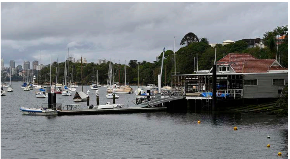
The rather naked boatshed on 5 May — ready for re-cladding
