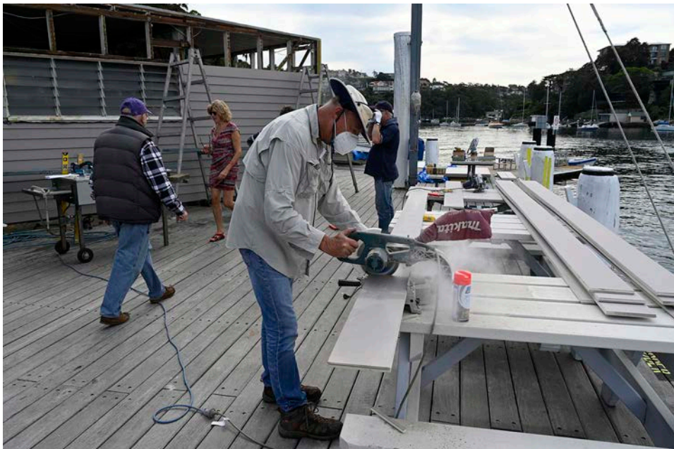
Peter Robinson cutting cladding to length on the wharf
