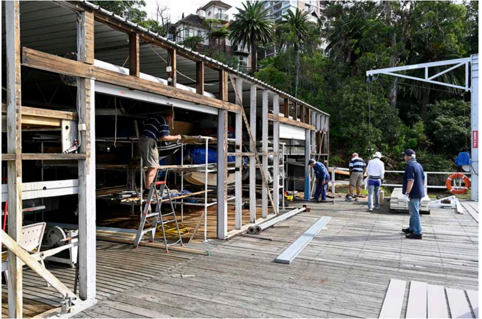
Work underway to reclad the boatshed on 8 May
