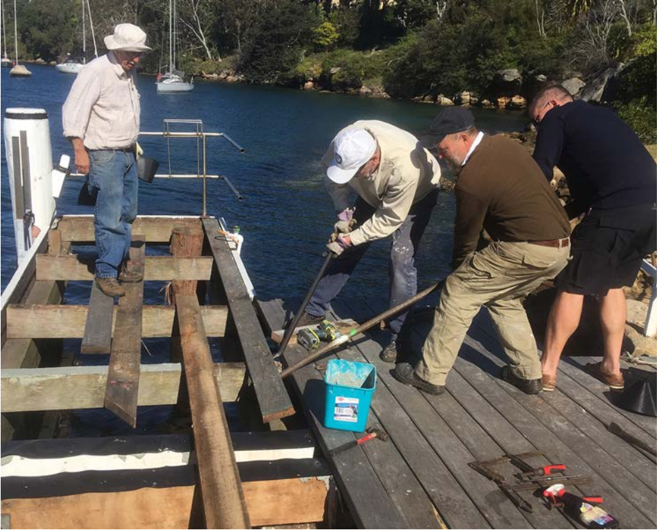
Muscle power and an old-fashioned crowbar lifted the old deck planks as willing volunteers got to work on the wharf on 25 July under the directions of the unstoppable Trevor Cosh
