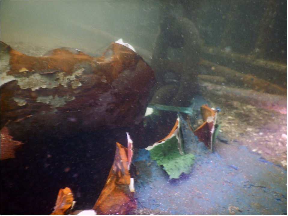
Chain cutting the accommodation block off
