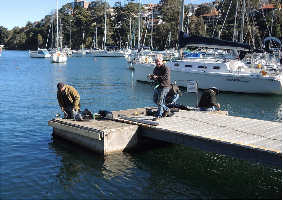
Fendering work underway on a pontoon at the Green Shed
