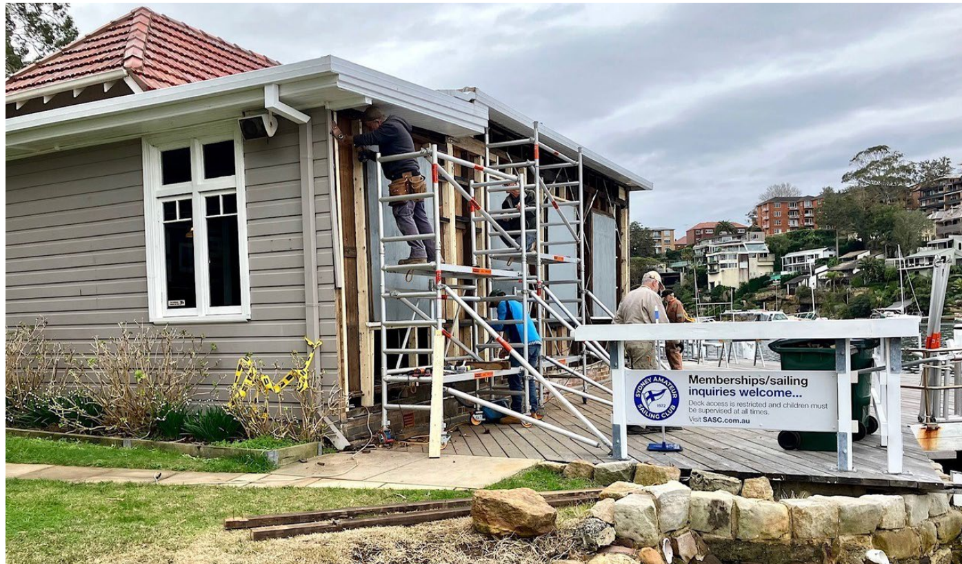
Photo: Demolition of the SE wall required scaffolding for safety
