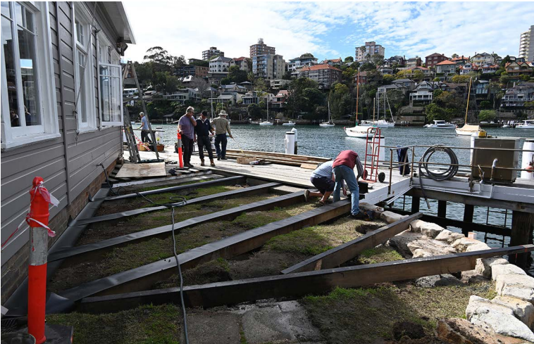
New deck beams completed
