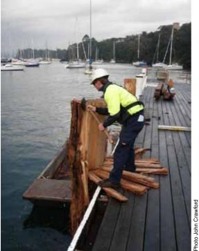
Placing a new free-standing pile off the SASC Wharf (above). Good progress was made in July on the repairs to the wharf and piles. The work should help hold everything together for a good few years to come
